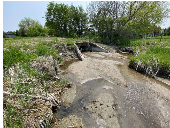
Photograph 20: WC1, upstream limits of watercourse feature at storm drain outlets (May 23, 2023).
