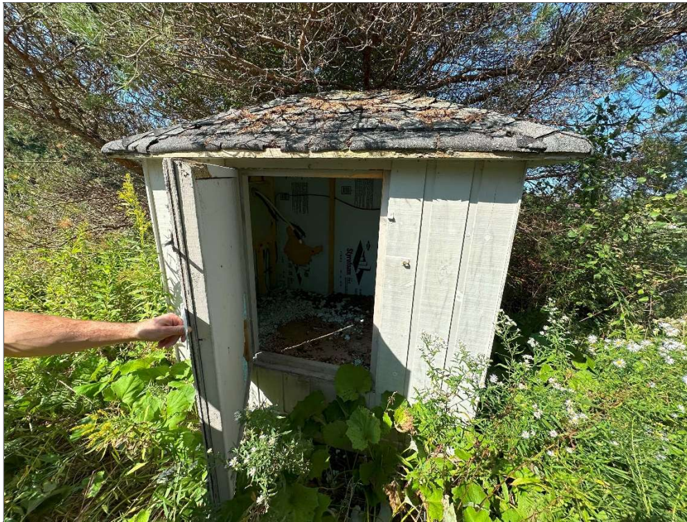
Photo 48 – Site Source water well house, view northwest.
