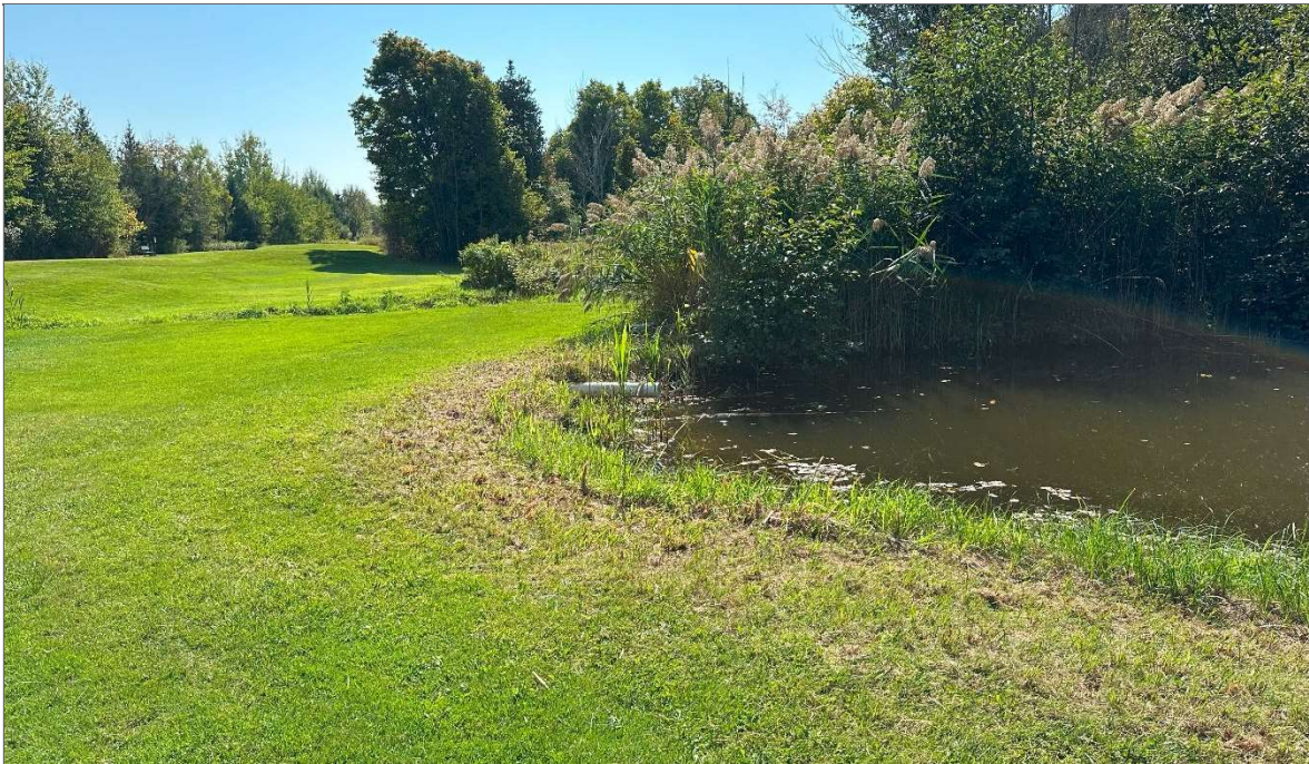
Photo 46 – French drain entering a waterhazard and silver creek at the north edge of the site, view south.
