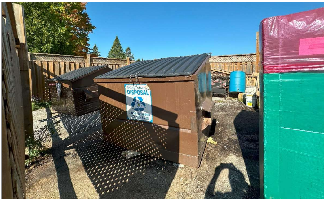
Photo 18 – Fenced waste management area northwest of the Clubhouse, view west.
