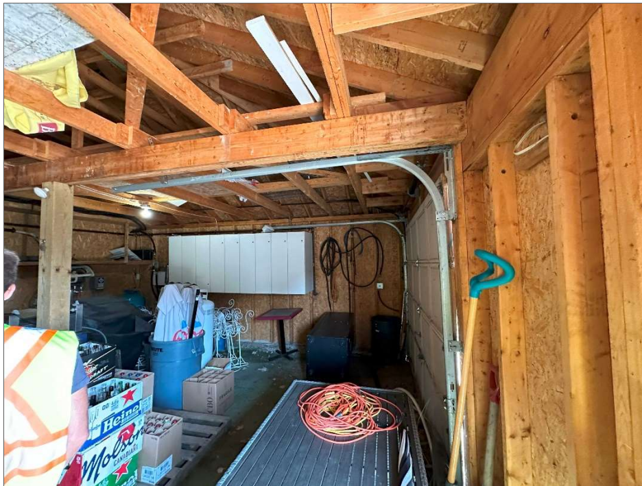
Photo 16 – Interior of the eastern end of the Grillhouse, looking northwest.
