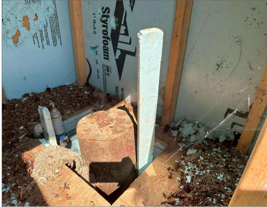
Photo 47 – Site source water well.
