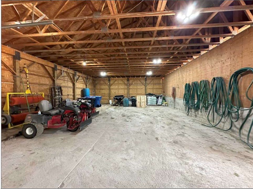
Photo 29 – Northeastern corner of the maintenance building, view northeast.
