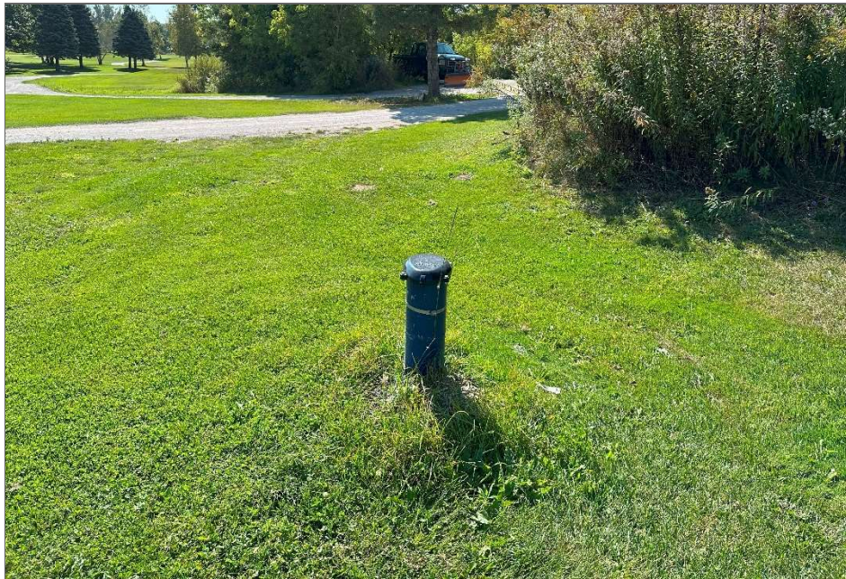
Photo 35 – Well located on the eastern side of the maintenance building.
