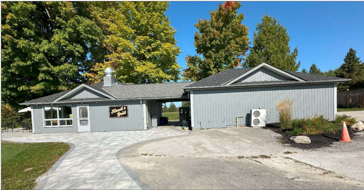
Photo 14 – Grillhouse building, view northwest.
