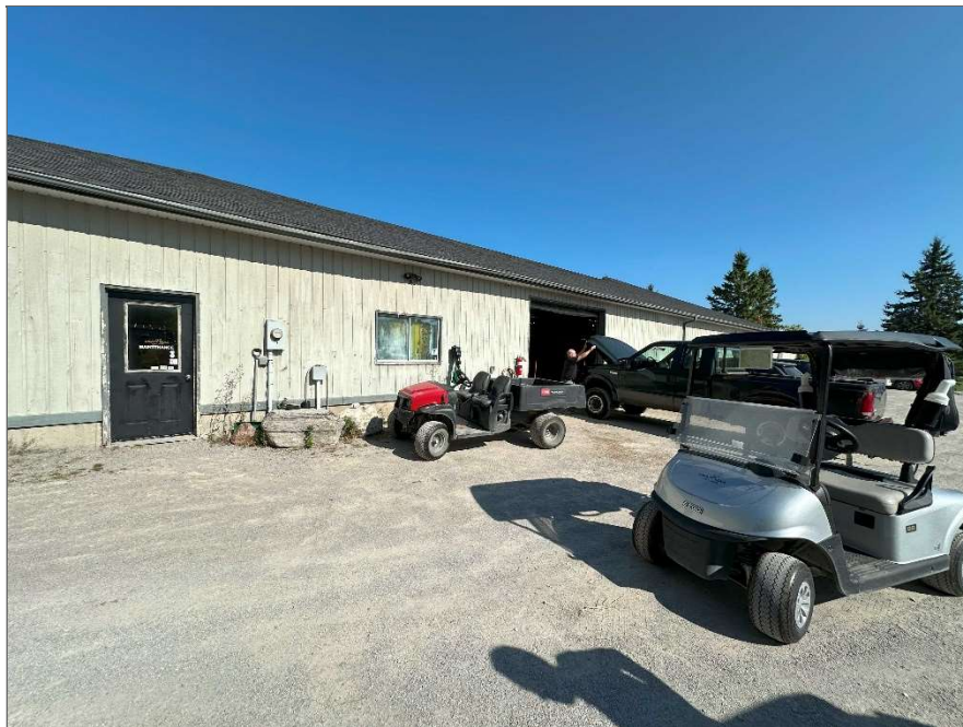
Photo 20 – Southeast side of the maintenance building, view north.
