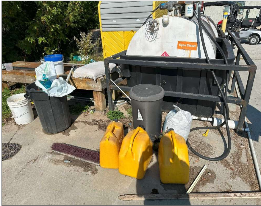
Photo 37 – Three (3) fuel storage containers in the spill capture area.
