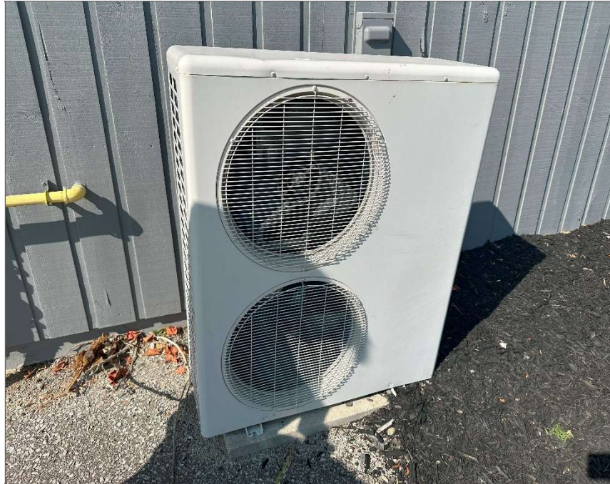
Photo 15 – Air conditioning unit located on the south side of the Grillhouse.
