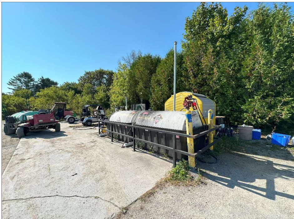
Photo 36 – Chemical use area located southwest of the maintenance building with spill capture drain, two (2) ASTs, and chemical waste storage bin, view south.
