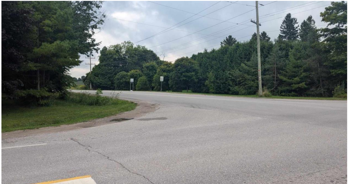
Division Road West looking southwest along Burnside Line. Drivers at the stop bar are unable to see more than 70 m when the plants have foliage.
