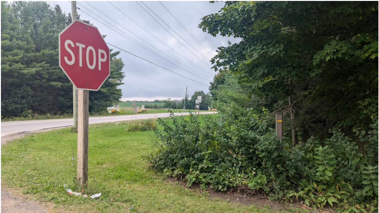
Division Road West looking southeast along Burnside Line. At the stop bar drivers can see approaching traffic from approximately 140 m.
