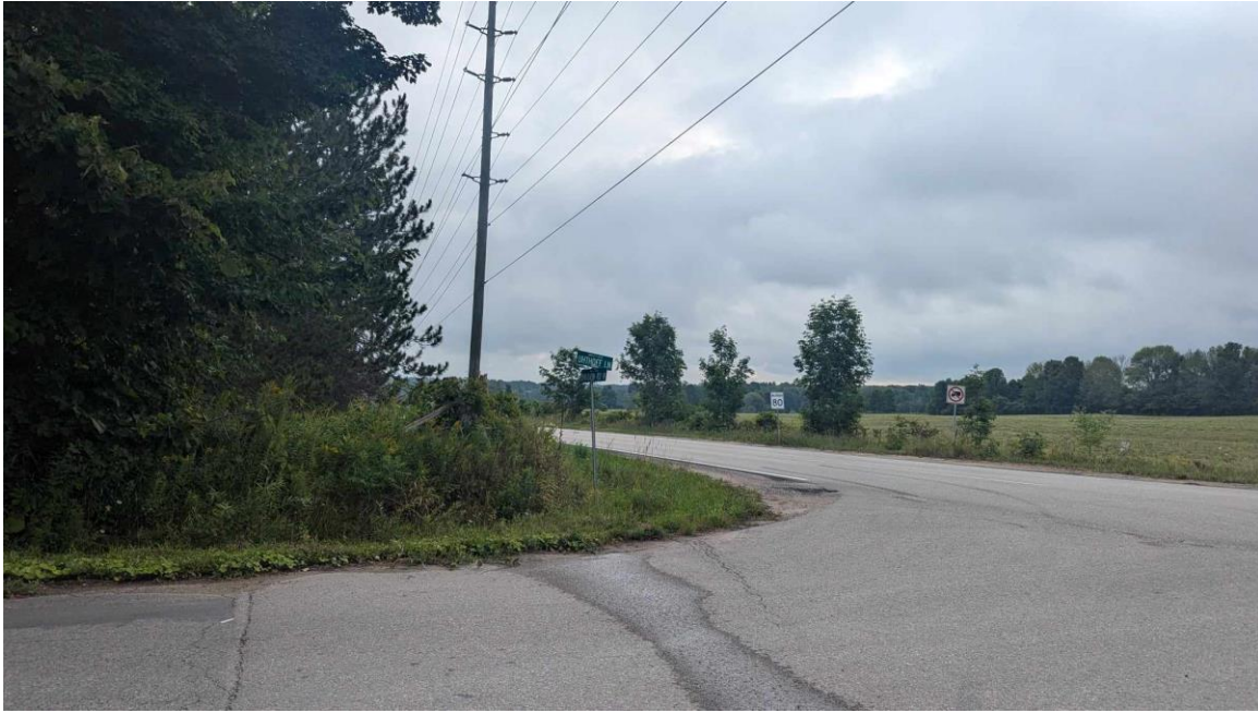
Uthoff Line looking southeast along Division Road West. Drivers at the stop bar are unable to see more than 30 m when the plants have foliage.
